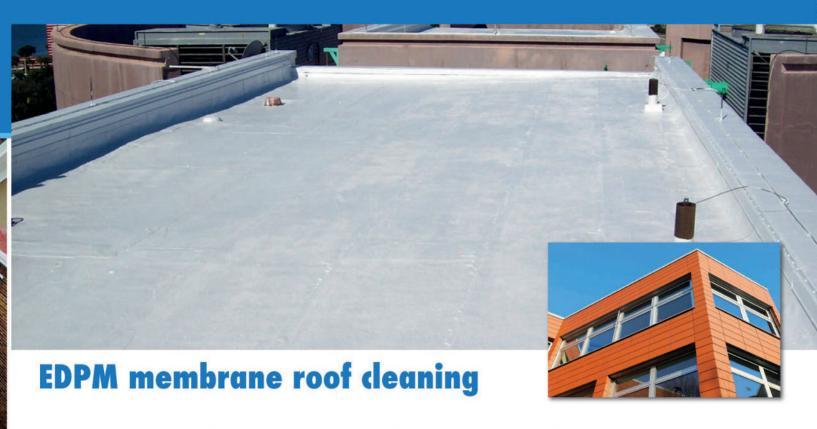
Flat roofs are usually light grey or white which reflects heat thus, keeping the building cooler inside. when molds, lichens, mildew and cyanabacterias are left to infest the EPDM membrane it does not take them too long to cover the roof in a dark colour, often greenish black in appearance.
