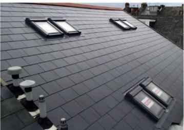
Many new builds now use fiber cement roof tiles. These offer a light weight, economical alternative to traditional natural roofing tiles. To prevent lasting damage occurring and costly repair costs they need to be protected.
